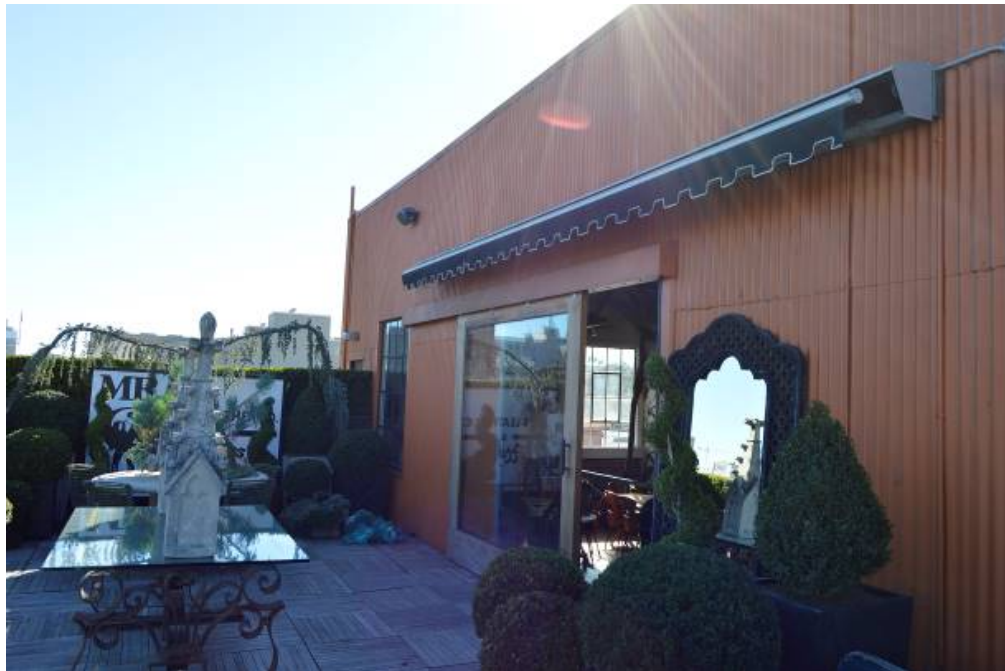
Figure 6: Third-story terrace and primary façade of 1927 addition. Fixed, steel-sash window in western bay not pictured. Looking southwest.
