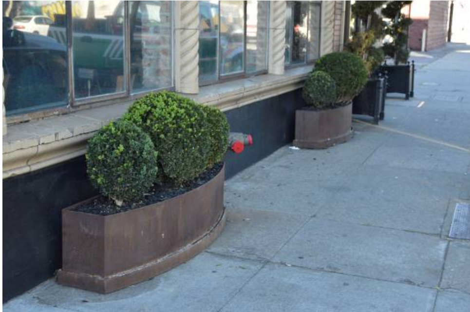
Figure 1: Original cement plaster water table, currently painted. Looking west.
