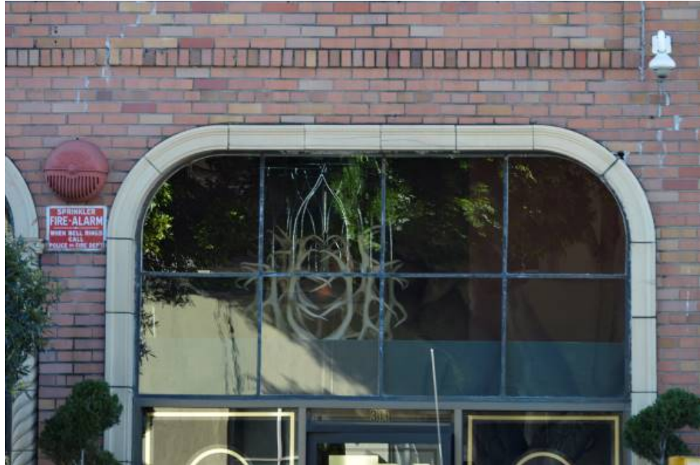
Figure 3: Divided-light transom above entry door in western bay, primary façade. Looking south.
