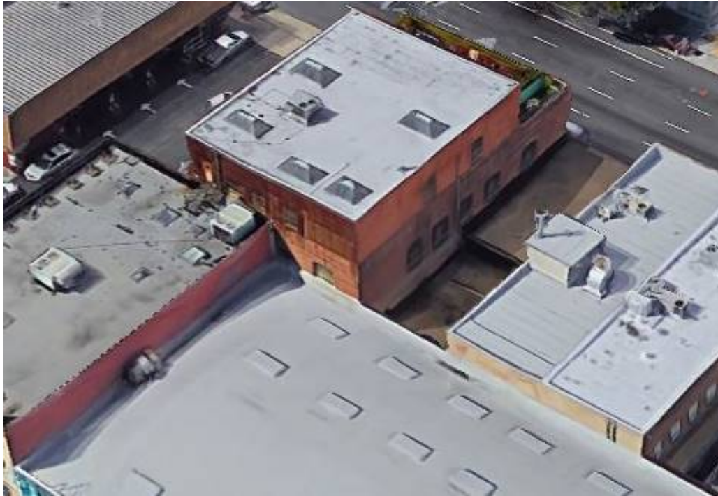
Figure 9: Aerial imagery shows rear façade of 310 7th Street. Looking north. Google Earth Pro, 2016. Edited by Page & Turnbull.
